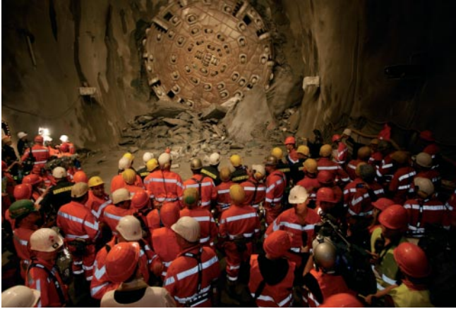
The mineure celebrate the break-through in the Gotthard Base Tunnel
