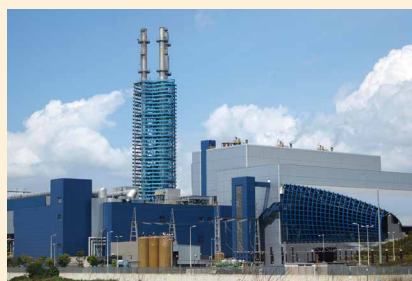
Waste incineration plant in Naples, Italy.
