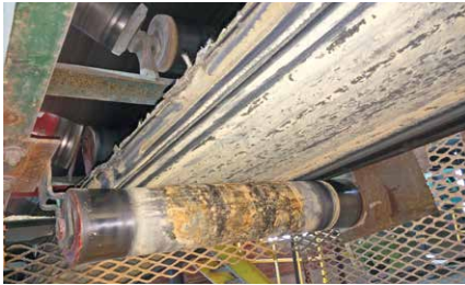
The belt conveyor before ...
